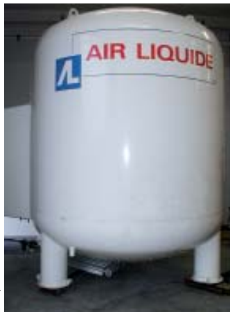
Nitrogen tank for the cooling system
